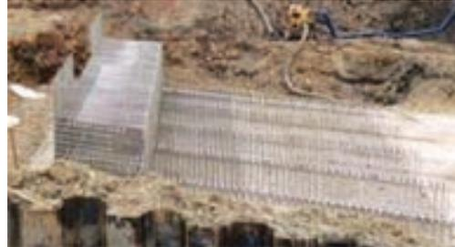
The Engineers also took into consideration the forgiving qualities of stainless steel. The concern about accurate translation of what is designed and specified in an office to actual practice on site can lead, for example, to lower than expected cover. A non-corroding form of reinforcement absorbs such variations thus avoiding future maintenance concerns.
